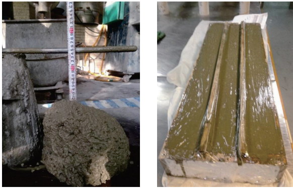
Fig. 3 Beams casting and fresh concrete performance.
