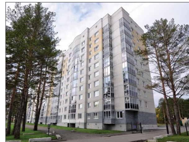
RESIDENTIAL COMPLEX ON THE MURANOVA STREET
