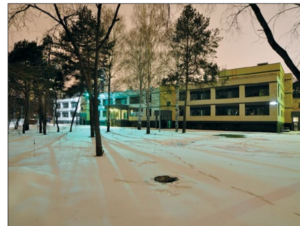
DIAGNOSTIC & TREATMENT COMPLEX
